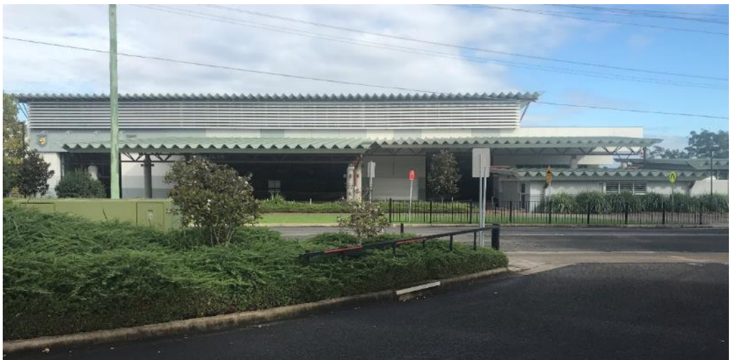
Figure 11 Sports Centre on Morris Grove
