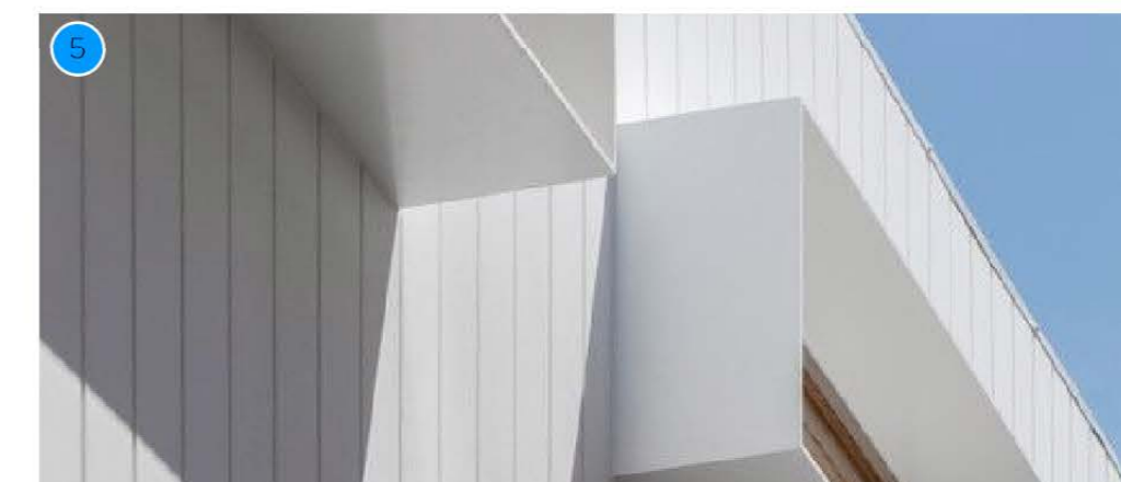
5. Light-toned profiled metal cladding to blend with sky and reduce visual impact of building mass
