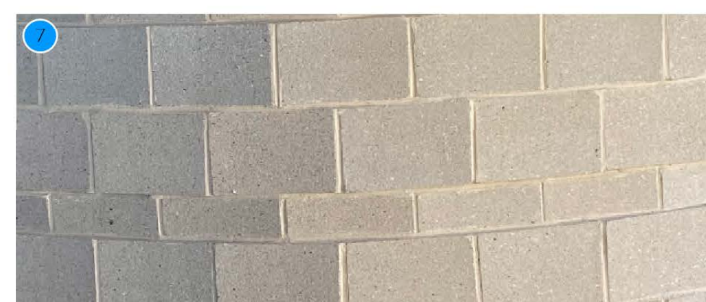
7. Sandstone blockwork to match newer buildings in the college.
