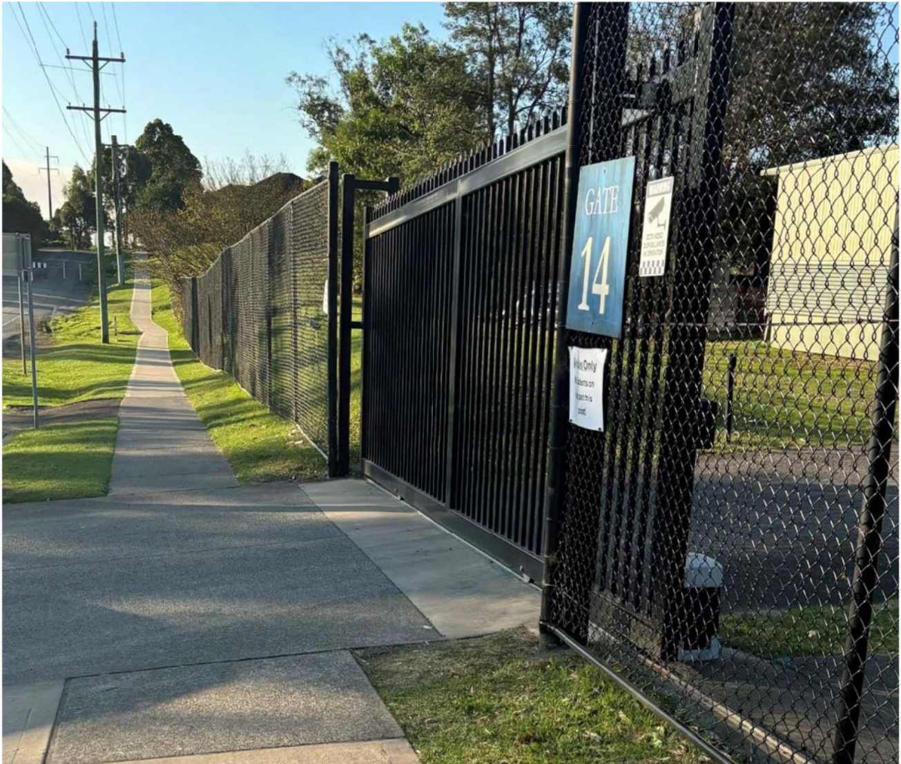
Figure 2.3 School access gate no 14 proposed for construction vehicle and construction staff access off Morris Grove
